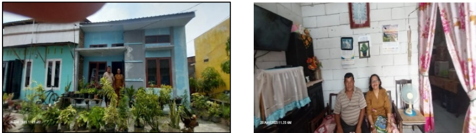
Figure 3. Satisfied beneficiary after house repairs
