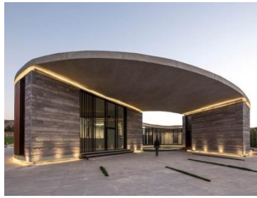
Gambar 6. This boutique dairy factory di western Turkey (diakses melalui : https://www.dezeen.com/2017/01/10/elliptical-dairy-factory-arkizon-slash-architects-turkey-wraps-around-outdoor-viewing-courtyard-cheese-showroom/ pada 17/01/2021 jam 4:35)
